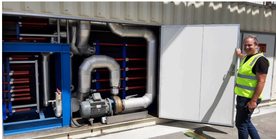
Adrian Finlayson shows part of the Brewery refrigeration system, using ammonia as refrigerant in an outdoor-located unit. The chill is transferred by heat exchanger to less-hazardous glycol for piped circulation through the plant
